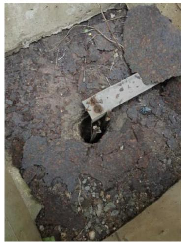
The second pit with the 2 driven rods. One rod is completely disconnected and the other rod seems to be partially connected to the copper busbar Date: 18/01/2022 Location: HSM
