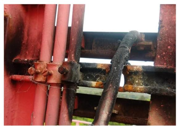
The DC armature cable going to the live rails behind. The cable has lost its Unistrut clamp allowing it to rub on the Unistrut rail
