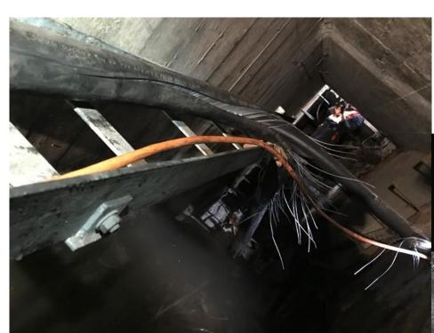
The scene inside the cable duct after the incident. Note the outer sheath of the XLPE cable has been cut back, the steel wired armour has been cut and pulled away from the cut site
