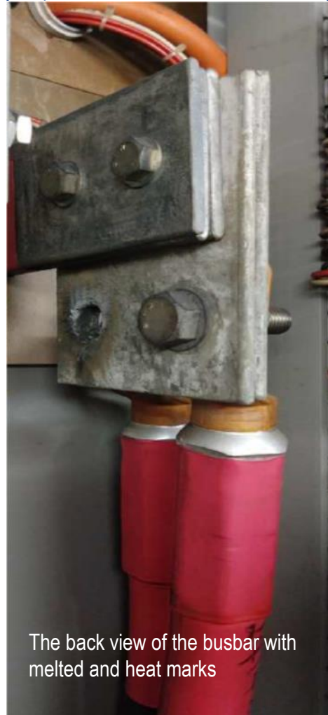
The bolted connection clearing open circuited from the busbar by the weigh of the cable and head of the bolt melting off
