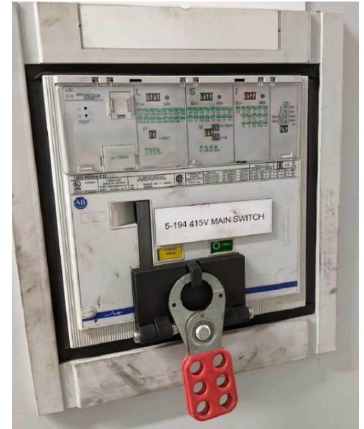
A metal jaw style multi-lock device presses the locking mechanism closer together ensuring the open pushbutton is sufficiently depressed to inhibit ACB operation
