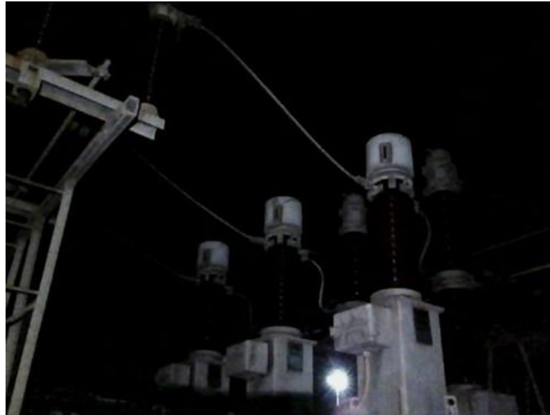
The incoming aerial supply CT connections at night when the hot joint occurred
