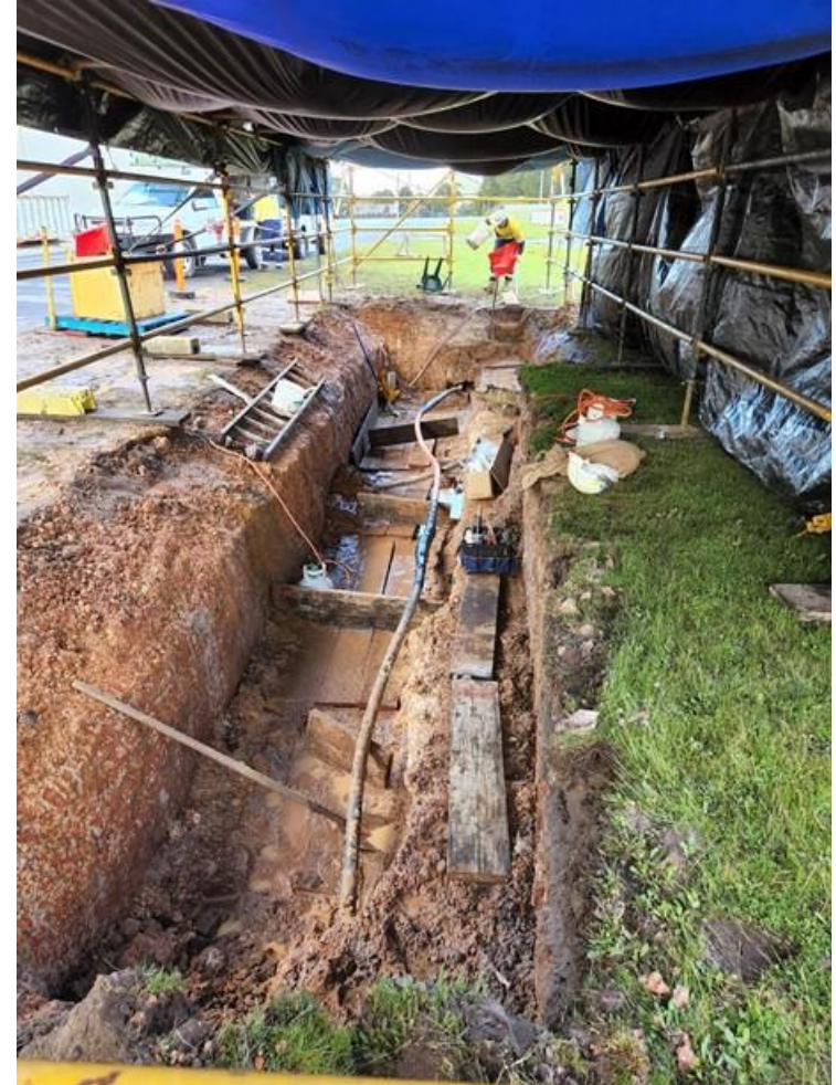
The excavation site of the new cable joints
