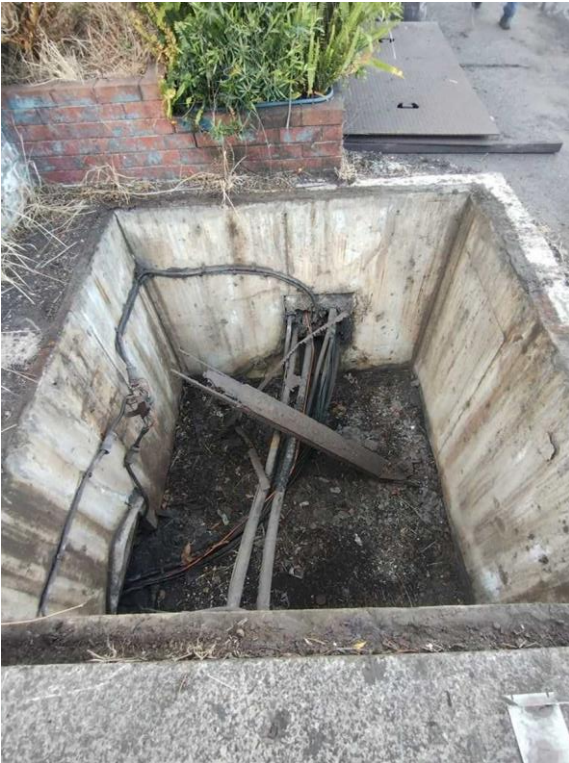
Pit with lid removed
