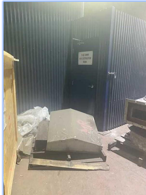
Switch room doors blocked by spares & trash – restricting access and emergency egress.
