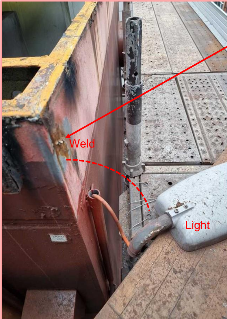
Light moved for scaffolding
